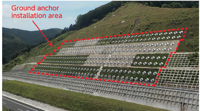
Photograph 1 Example of a slope with ground anchors installed
