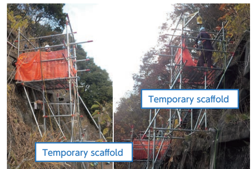
Photograph 3 Example of a temporary scaffold
